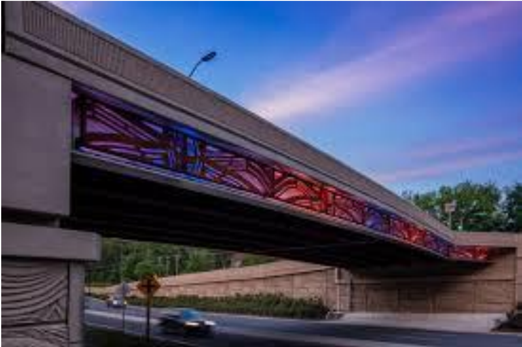
Arlington Bridge Route 50 Vicki Scuri Arlington, VA
